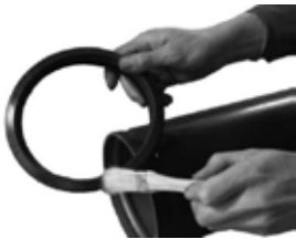
2.Lubricate gasket Check gasket to be sure it's compatible for the intended service. Apply thin lubricant to the outside and sealing lips of the gasket.
