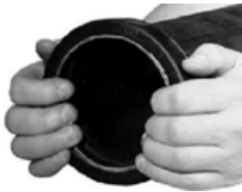
3.Gasket installation Slip the gasket over one pipe, making sure the gasket lip does not over-hang the pipe end.
