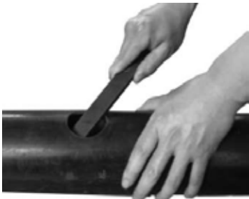
2.Remove burrs If any burrs or slug exists at the pipe hole, please remove them before assembly, to protect the gasket and avoid leakage.
