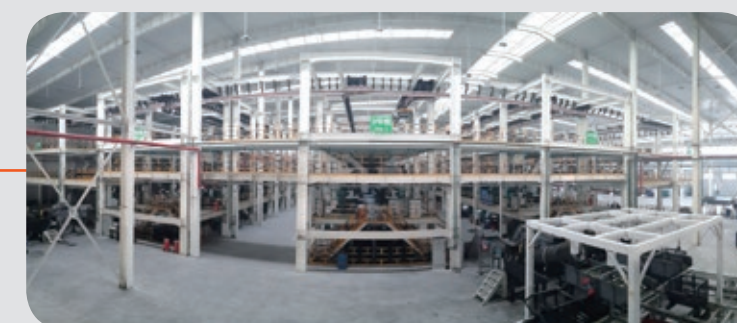
Threading, Air Pressure Test, and Anti-rust Treatment
