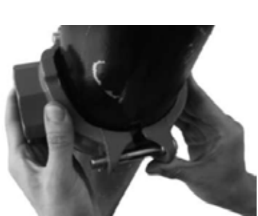
4.Alignment Align the strap around the pipe, insert the bolts and tighten the nuts finger tight.
